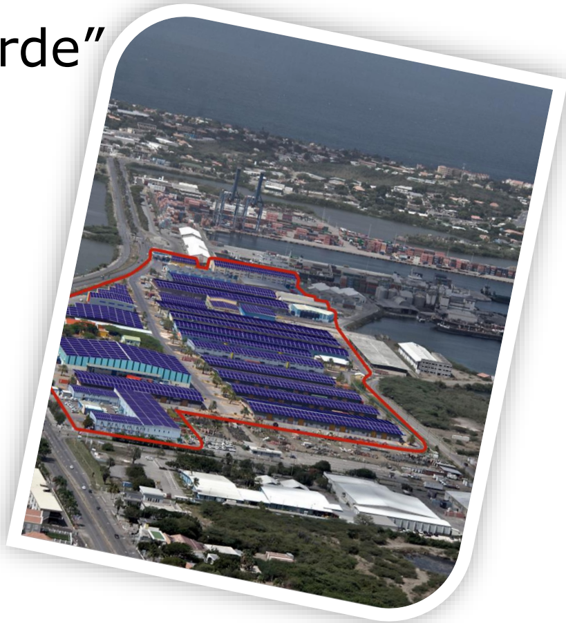
20 MW Rooftop Solar park
